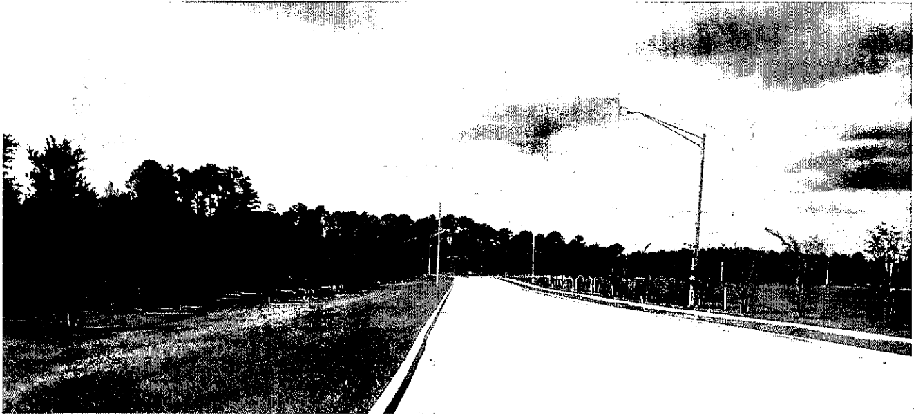
The subject site on the left facing northwest along R.G. Skinner Pkwy.
